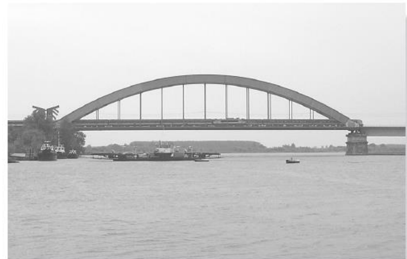
Arches support their loads in compression.
